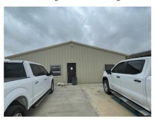
East Side Rear: Remove and replace approximately 50ft of 4in gutter, remove and replace one 10ft downspout. Remove and replace approximately 30sqft of soffit. Color match existing
